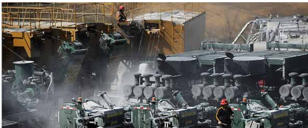
Typical equipment on a horizontal gas well site (Photo: catskillmountainkeeper.org)
